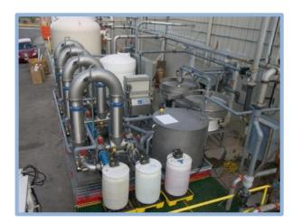
**Technology** – The design objective is to clean reclaimed graywater to specification for reintroduction into the intake of the entire wash wheel without adversely affecting chemical addition, product quality or laundry system operation. These design goals also use only the latest filter and advanced oxidation technologies on the market.
