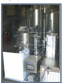
water then flows through 25 micron tubular prefilter and on the ultrafilters. The final stage is complete disinfection in anultraviolet chamber making the treated wastewater suitable for recycling or beneficial reuse.
