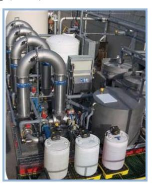
level. The final stage is complete disinfection in a ultraviolet chamber. Treated wastewater may then be discharged, recycled or reused.
