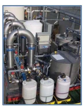
level. The final stage is complete disinfection in an ultraviolet chamber. Treated wastewater may then be discharged, recycled or reused.
